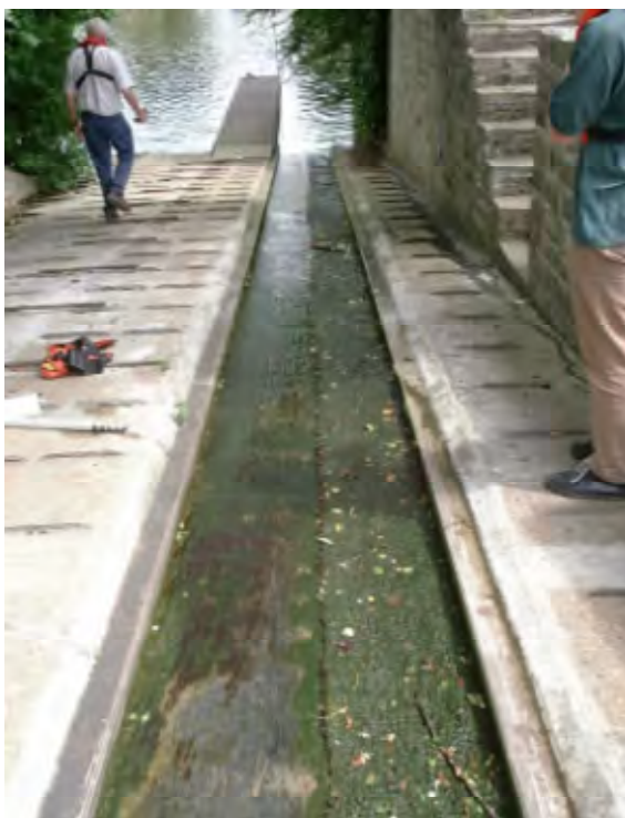
Figure 4.2.11 Canoe ramp at Sunbury lock showing Enkamat elver substrate on right-hand side.
