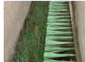
Figure 4.3.12. Detail of the substrate in the Plancoet Dam pass
