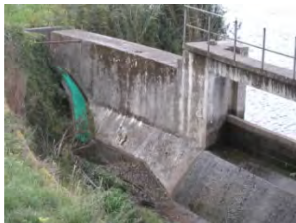
Figure 4.3.2. Pont Avet elver pass.
