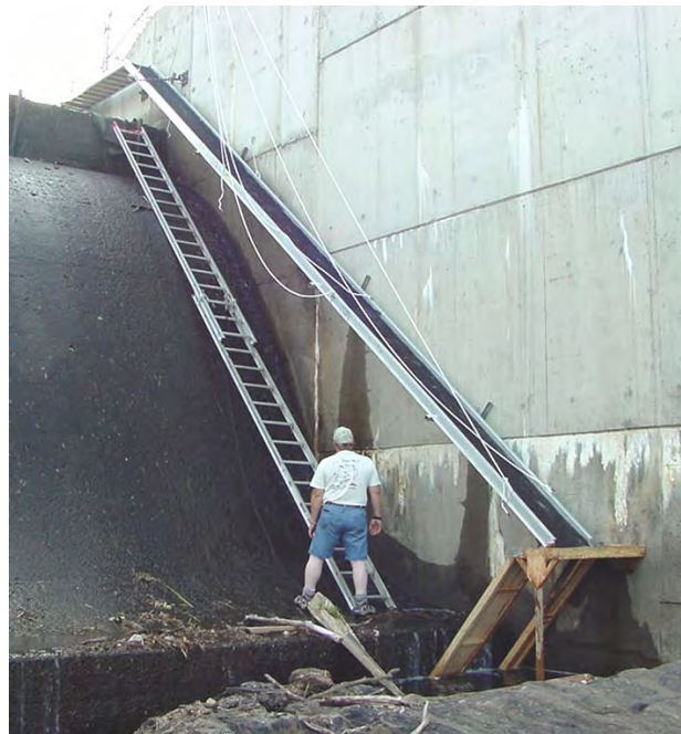
Figure 4.4.9. Pass at Benton Fall Dam. Note layout to ensure entrances to pass are close to the dam face. Photo G Wippelhauser
