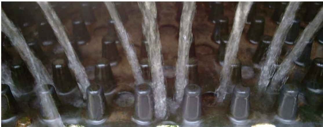
Figure 4.4.16 Top of one of the ramps at the Westfield pass-trap showing the Akwadrain substrate and the jets of water irrigating the ramp.
