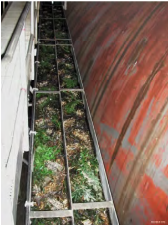
Figure 4.4.2. Details of the double channel pass at Moses-Saunders Dam. Photo D. Desrochers
