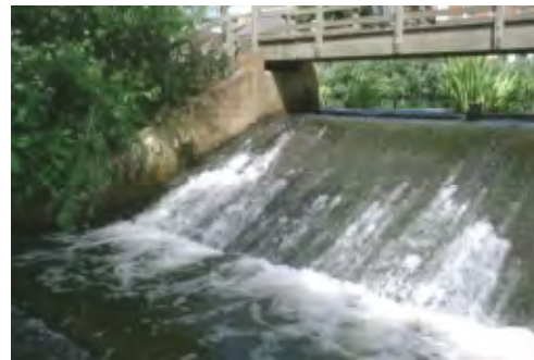
Figure 4.2.16. Cobham Mill Weir. Note vertical lip at weir crest, and broken water due to roughened surface.
