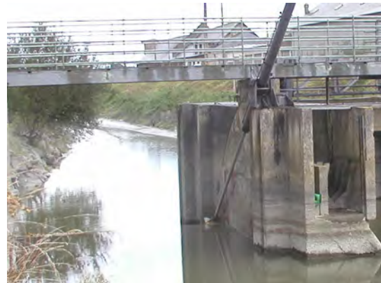
Figure 4.3.11. Plancoet Dam from upstream. The sluice is open so the water surface is well below the usual retained level.
