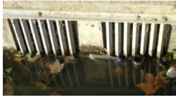
Figure 4.3.22. Trash screen at the upstream end of eel pass at Rennes Weir
