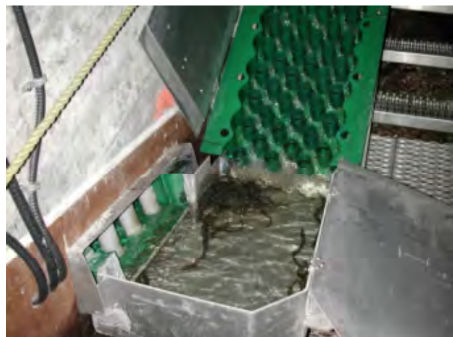
Figure 4.4.6. The bend between Sections 3 and 4 of the new eel pass at Beauharnois. The aluminium lids are lifted to show the ‘Eel-ladder’ substrate and the resting chamber. Many small eels are visible in the resting chamber. Photo D. Desrochers
