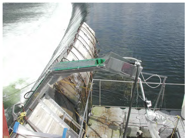
Figure 4.4.4. View of Chambly Dam eel pass from above. Note breakwater blocks on dam crest, covers over the channel containing “Eel – ladder” substrate, and electronic counting device on the pipe carrying the eels from the top of the pass to the keep net with its flotation collar. Photo D. Desrochers
