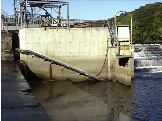
Figure 4.4.13. Eel pass at Greenville Dam. Photo A. Haro
