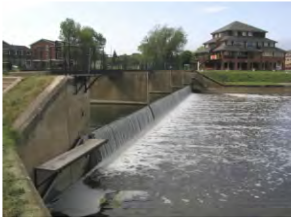
Figure 4.2.3 Elver passes at Stanchard Pit Weir
