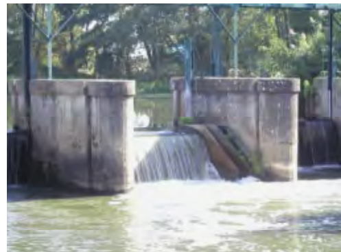
Figure 4.3.18. Eel pass at Moulin a Pigné
