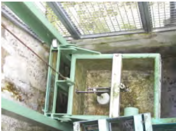
Figure 4.3.14. Lift hopper at Ville Hatte Dam eel pass in lower level position.
