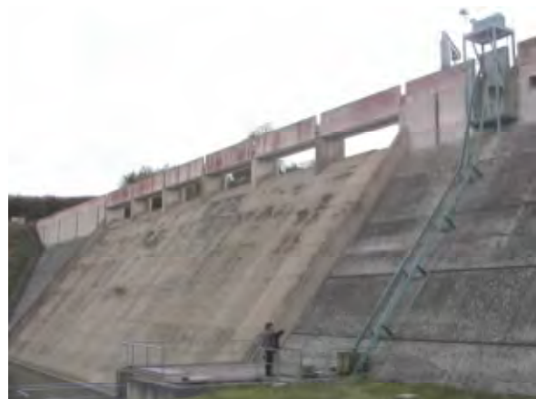
Figure 4.3.7. Eel lift at Bois Joli Dam.
