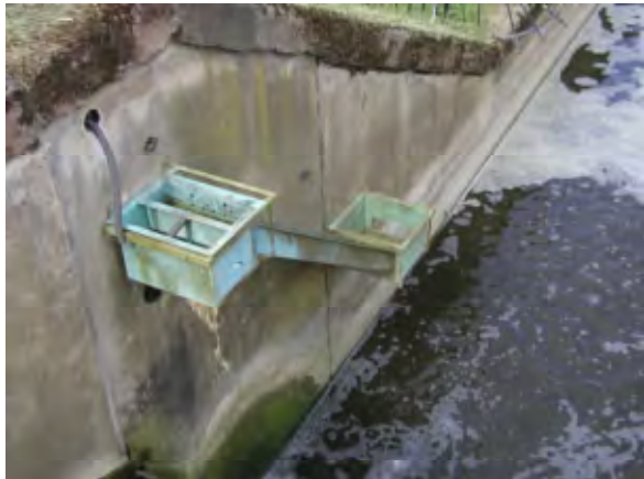
Figure 4.2.4 Left-bank elver pass at Stanchard Pit, with lower ramp missing due to flood damage.
