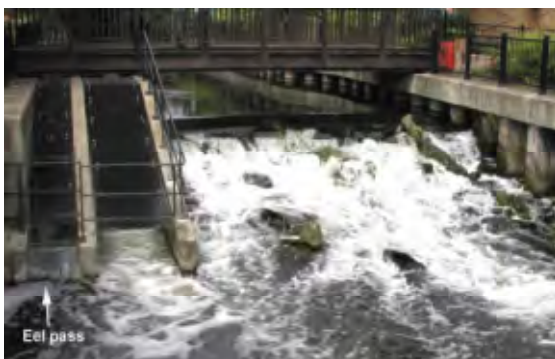
Figure 4.2.19. Staines Lino Mill eel and baffle passes.
