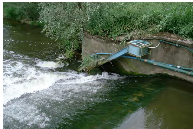
Figure 4.2.7 Right-bank eel pass at Strensham Weir. It has been severely damaged during a flood by a log that is still jammed beneath the resting pool.
