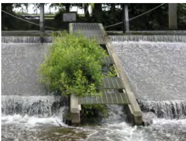
Figure 4.2.12. Sunbury Weir elver pass
