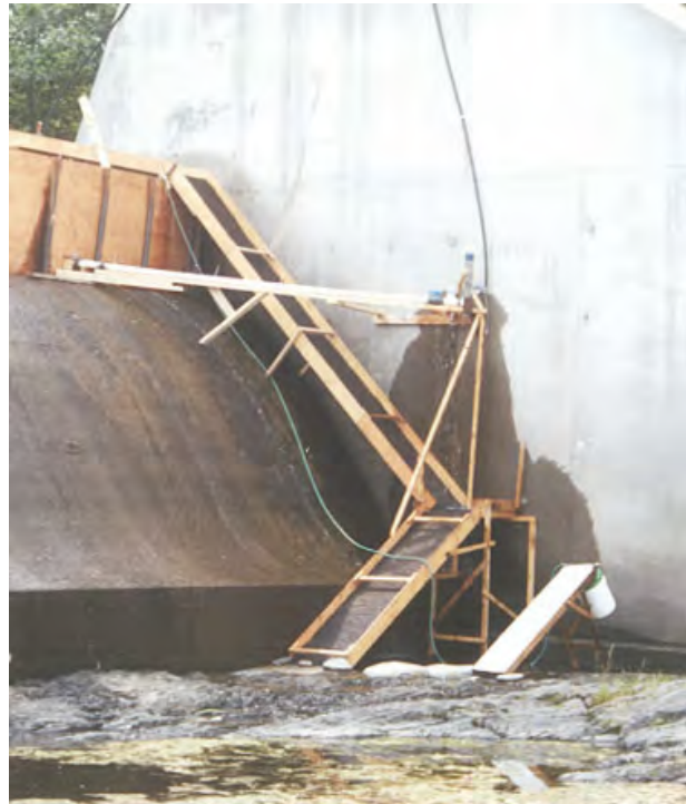
Figure 4.4.8 Pass at Fort Halifax Dam. A “portable passage” ramp is being deployed alongside. Note layout to ensure that entrance to pass is close to the face of the dam. Photo G Wippelhauser
