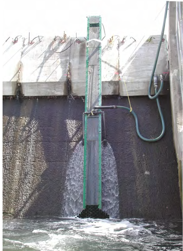
Figure 4.4.3. Eel pass at Chambly Dam. Note the breakwater blocks on the dam crest, and the gravity-fed attraction water being discharged from two pipes part way down the dam face. Photo D. Desrochers
