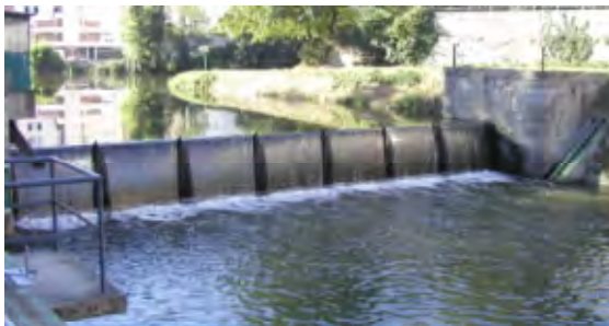
Figure 4.3.20. Eel pass at Rennes Weir
