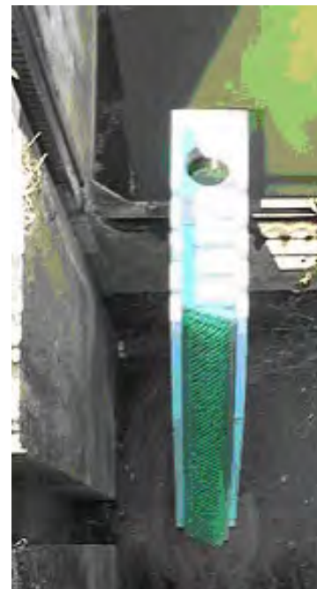
Figure 4.3.24. “Fish-Pass” prefabricated sluice gate pass
