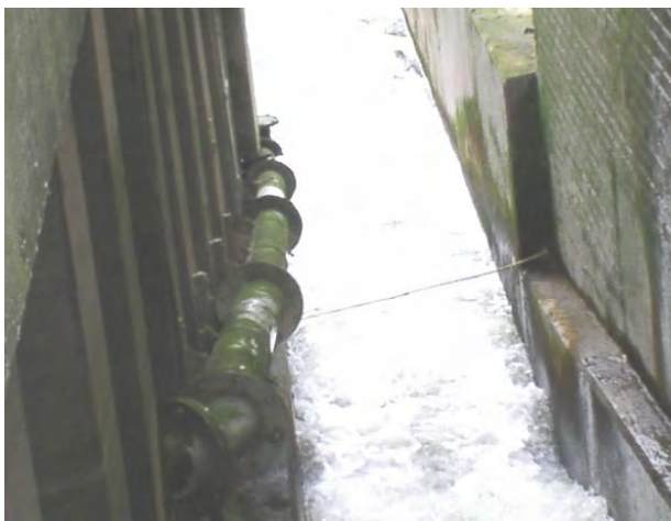
Figure 4.2.21. View down the fish pass at Barking Barrage at low tide. The elver pipe pass is on the left, and passes through the wall of the fish pass. The top of the perforated vertical stand pipe that represents the entrance of the pipe pass is just visible at the far end.
