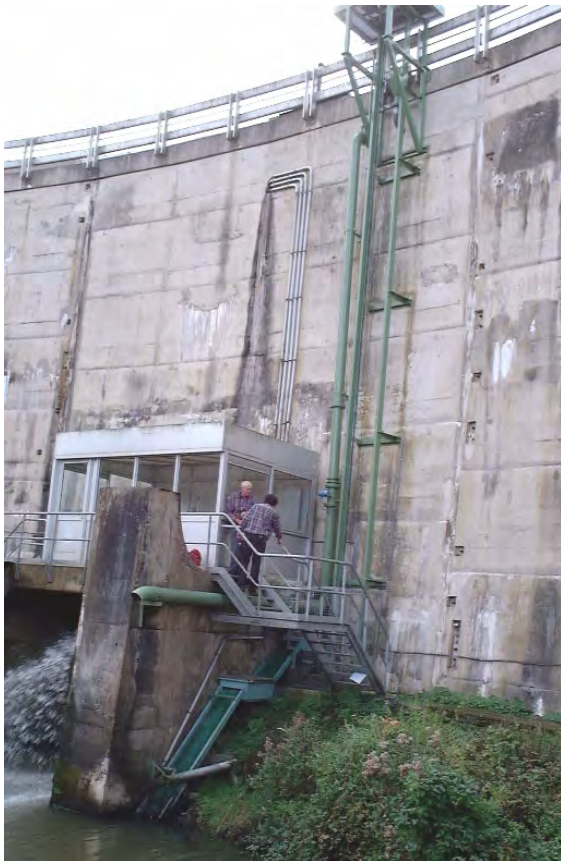
Figure 4.3.13. The Ville Hatte Dam eel lift. The substrate ramps can be seen below the platform.
