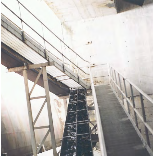
Figure 4.4.1. Two ramps of the new double-channel Moses-Saunders eel ladder. Photo D. Desrochers.
